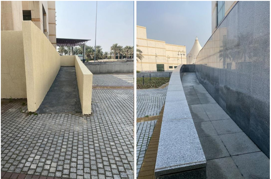
(Figure 4) Images of sample ramps of the college building (Images by Author)
